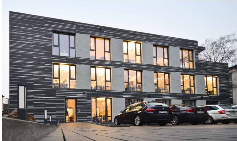
Exterior view of the extension of the HAMBORNER administrative building
